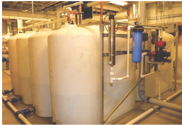
Rain System (Barr Plastics Photo)
